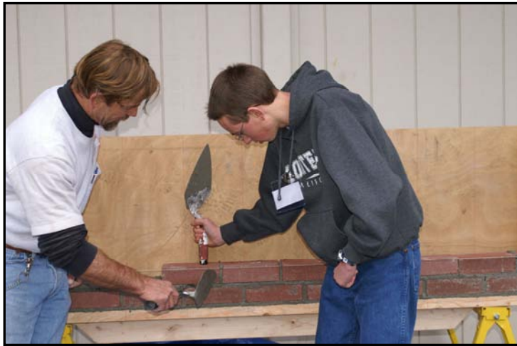
Eric Anderson, from the Bricklayer Local Union, helps Galt High School student Matthew Hunt secure his brick properly.
