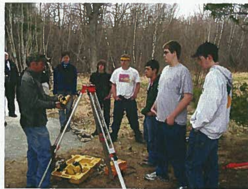
UTC Technology Instructor John Milligan discuss the correct techniques associated with operating a laser level and transit during an actual project in which ACE students constructed a pathway..
