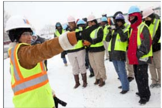
Lisa Anders, senior project manager for the Martin Luther King, Jr. National Memorial, leads a tour of the memorial construction site.
